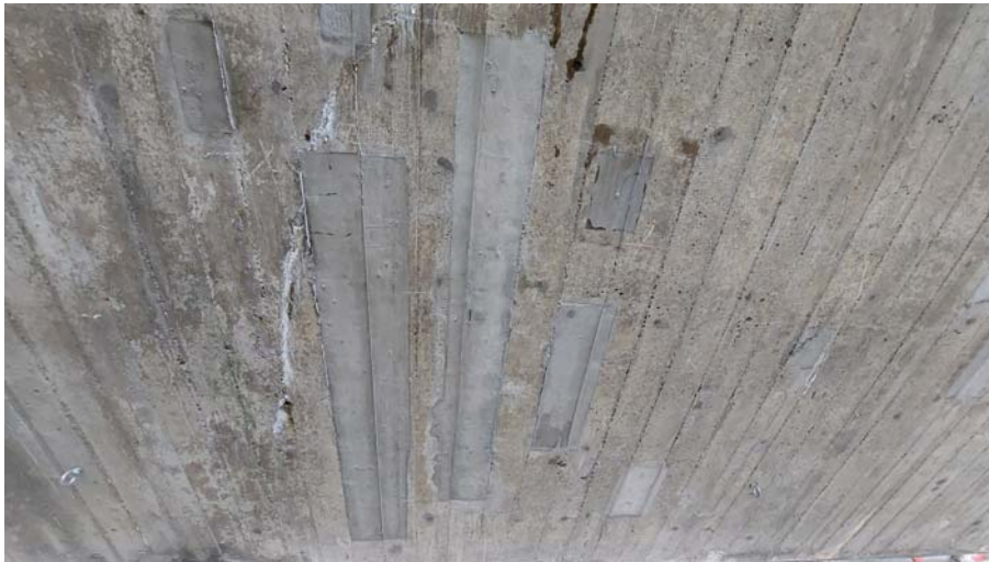
LEFT: Figure 5 – trial repairs carried out to the underside of the roof.
